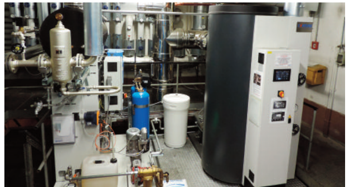
CERTUSS Universal 850 TC, natural gas, with CVE supply unit
